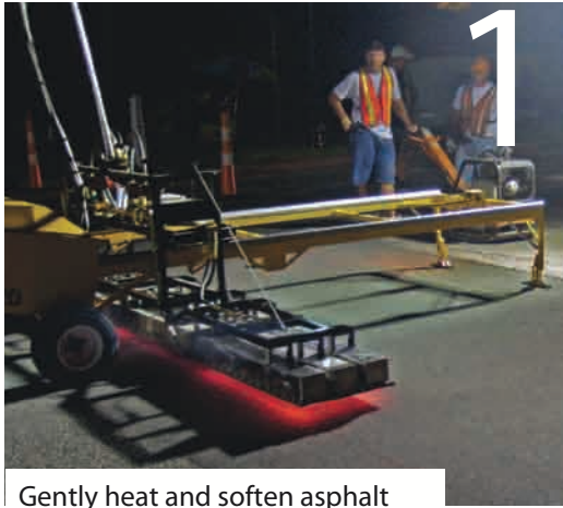
Gently heat and soften asphalt
